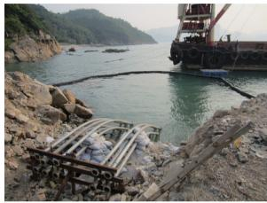
Photo 1 - A silt curtain was employed around the seawall area.
