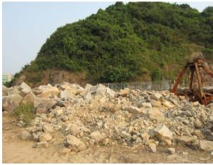
**Photo 3 -** Tarpaulin sheets to cover dusty stockpiles to prevent dust generation were absent from the construction site.
